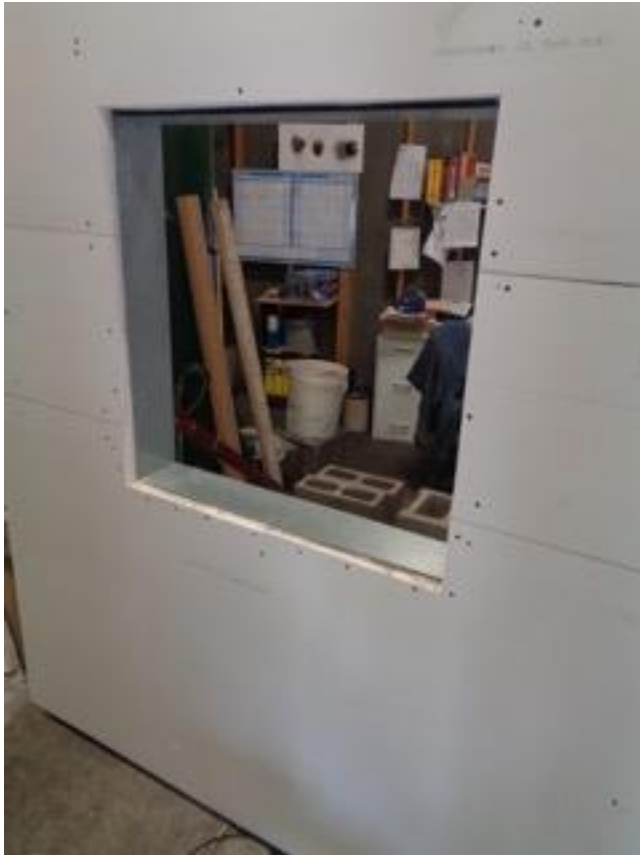
Wall construction, exposed side
