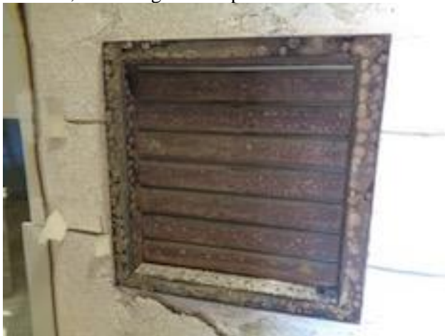
Post test: Exposed side of test sample
