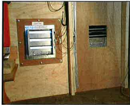
Photo 2 of FM200 Positive Pressure Vent Opening (Bottom blade locked shut) →
